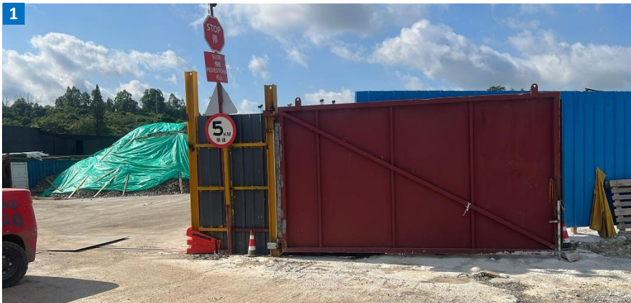
"5KM/H" signs erected on both sides of the site access.
